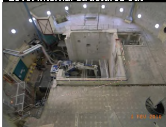
2010: Internal structures out
