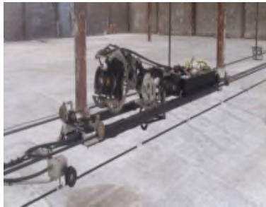
In concrete structures
