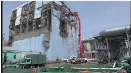
Water discharge to spent fuel by concrete pump car
