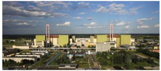
4 VVER-440 type Units; Commissioning time: 1982-1987 Original design: 1375 MW, 440 MWe, After power uprate project 1435 MW, 500 MWe
