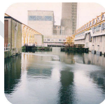
Figure 1: Sellafield Local Effluent Treatment Plant
