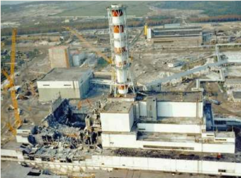
Reactor building immediately after the accident
