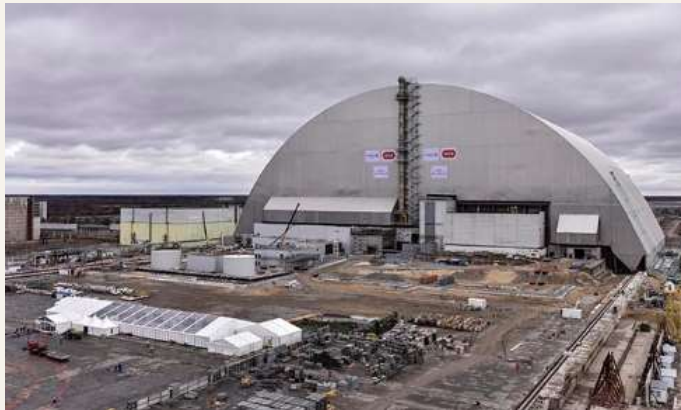
New shelter (installed November 2016)
