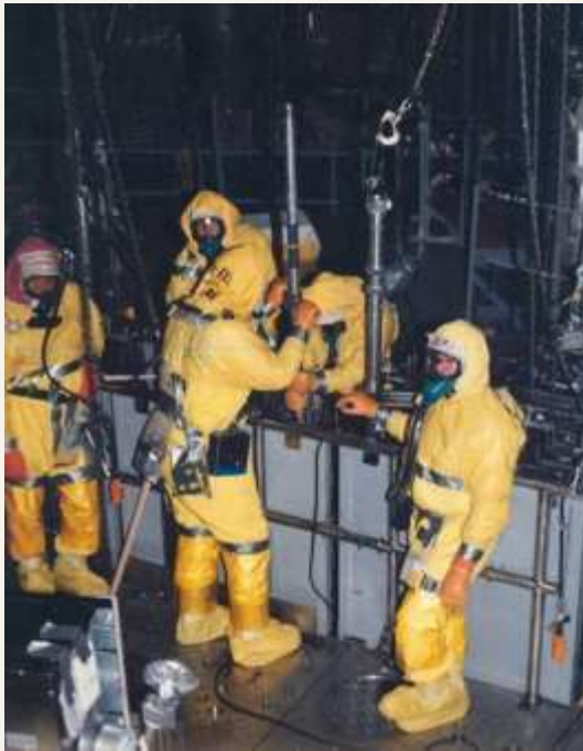
Work over the reactor core
