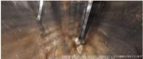
The bottom of the Unit 2 PCV (photo taken by remote-camera)
