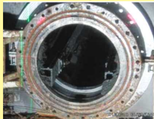
Removal of deposits completed
