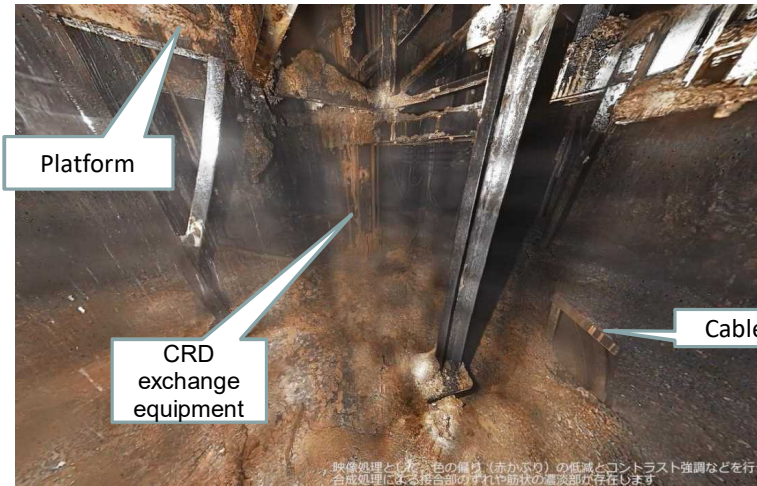
Example of equipment layout in Mark-I containment vessel
