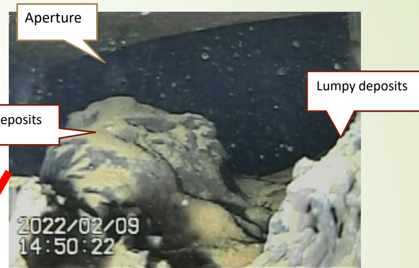
B. Inside the pedestal opening Lumpy deposits
