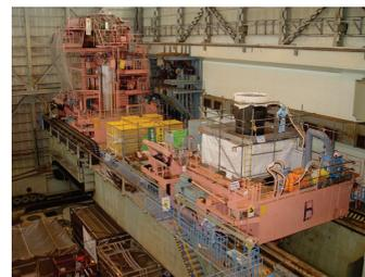
Figure 1. Dismantling of Fuel handling Machine
