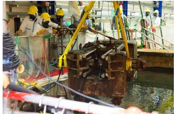
Figure 1. Removal of waste from a Sellafield Pond
